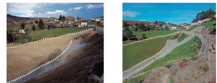
Figure 12: the before and after of ecological restoration via revegetation with local species of an embankment affected by landslides using the ECOVARS approach, in Gazost, Midi-Pyrénées. Source: CBNPMP
